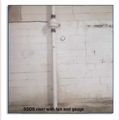
the warehouse floor and sealed to the top of the floor. Special attention was made to the placement of the eight vertical PVC pipes so that useable warehouse space was not lost. To minimize the impact to the warehouse footprint space, the SSDS pipes were installed in horizontal trenches below ground until they transitioned to vertical SSDS piping.
