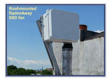
dition resulted in a necessary modification in system design to substitute a RadonAway fan in place of the originally-specified FanTech fan. The RadonAway Fan was preferred as it will induce greater air flow to the vacuum pits with little increase in vacuum.
