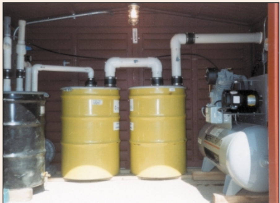
Figure 6. A typical soil vapor extraction and air sparging system used at dry cleaning facilities.
