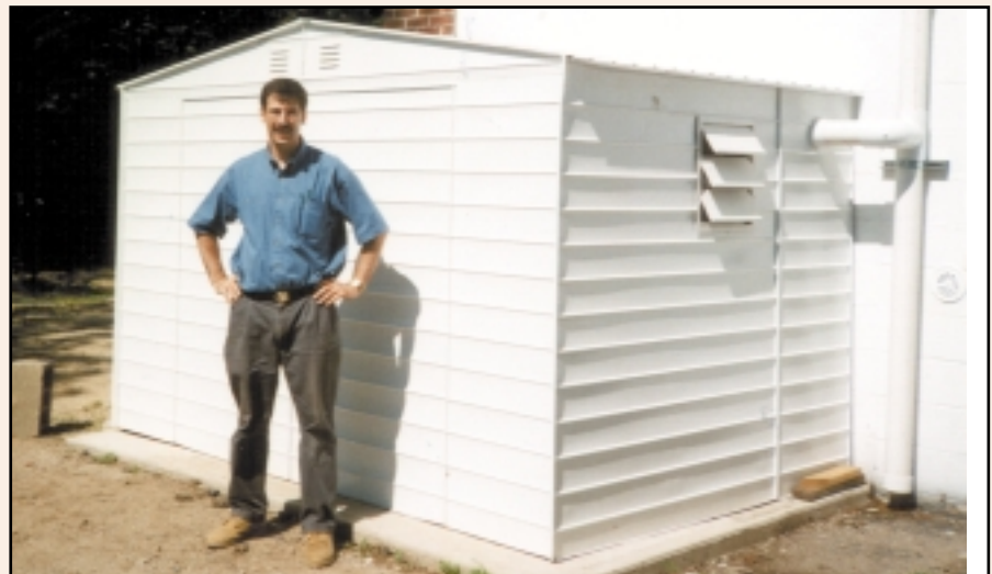
Figure 5 - Equipment shed used to house a soil vapor extraction and air sparging system located behind a dry cleaning facility.
