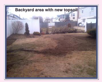
Endpoint sample results confirmed successful removal of all contaminated soils. Clean topsoil was then brought in to fill in the excavated areas. Upon completion of the topsoil placement, a Report was prepared and submitted to NYSDEC for Spill Closure on behalf of the homeowner.
